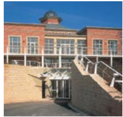
Location: Hawkstone Park Golf Course Architect: The Sir Basil Spence Partnership (now known as Blee Eitwein Bridges) Fabricator: Armston Ltd, Newcastle
